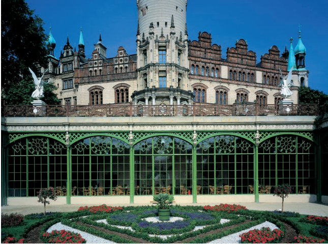
Orangery Schwerin Castle, Schwerin, Germany
