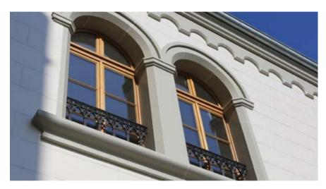
The windows have a rounded "Wolfsrachen" closure design and were faithfully reproduced using SCHOTT RESTOVER®. Thin panes of insulating glass provide the necessary heat insulation. A final detail in recreating the windows was replicating the espagnolette window locking devices.
