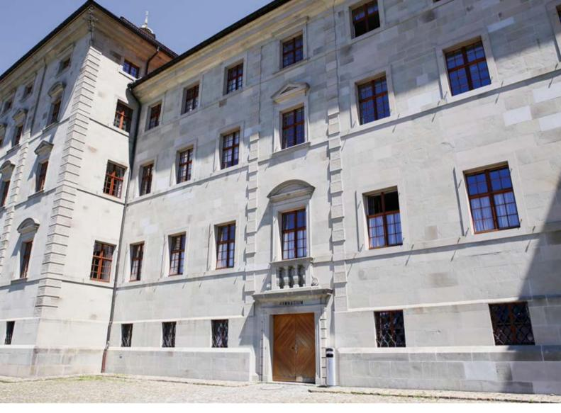
Full restoration is taking place from 2013 to 2022 and aims to recreate the original Baroque appearance which to some extent had been distorted by earlier renovations. The new renovation uses SCHOTTTIKANA® in the main exterior of the Einsiedeln Abbey. The glass has a slightly irregular surface to blend harmoniously into the overall image, and combines a historical look with modern building properties.
