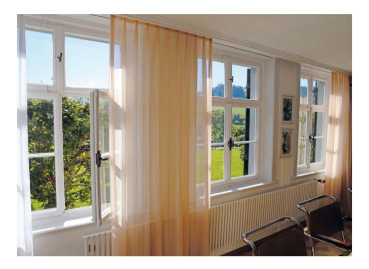
RESTOVER® reproduces window glass manufactured around the turn of the century. Its reduced thickness enables easy installation in historical window frames and profiles.
