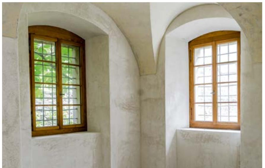
Restored using SCHOTT RESTOVER®, frames made from oiled chestnut wood
