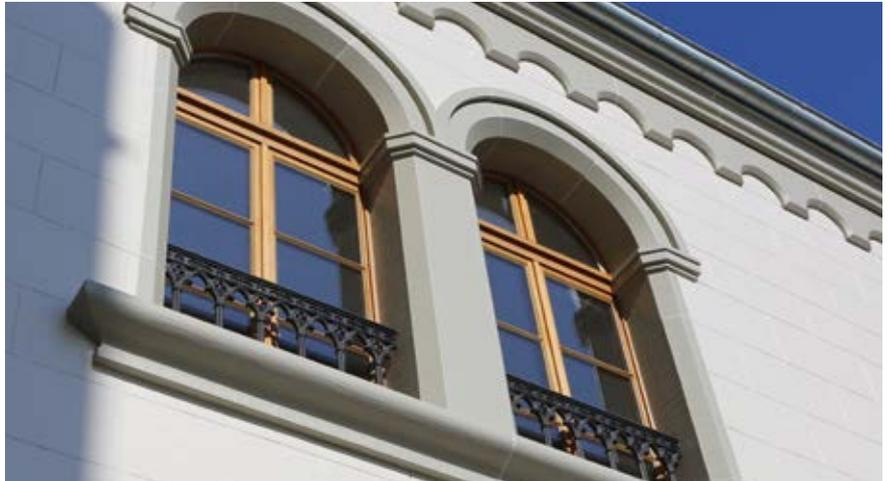
The windows have a rounded “Wolfsrachen” closure design and were faithfully reproduced using SCHOTT RESTOVER®. Thin panes of insulating glass provide the necessary heat insulation. A final detail in recreating the windows was replicating the espagnolette window locking devices.
