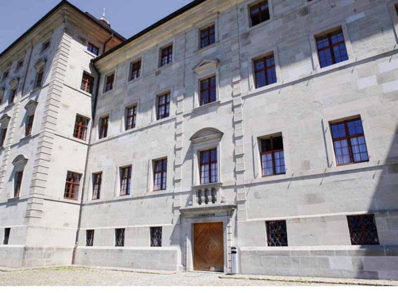
Full restoration is taking place from 2013 to 2022 and aims to recreate the original Baroque appearance which to some extent had been distorted by earlier renovations. The new renovation uses SCHOTTTIKANA® restoration glass in the main exterior of the Einsiedeln Abbey. The glass has a slightly irregular surface to blend harmoniously into the overall image, and combines a historical look with modern building properties.
