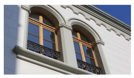
The windows have a rounded "Wolfsrachen" closure design and were faithfully reproduced using SCHOTT RESTOVER® restoration glass. Thin panes of insulating glass provide the necessary heat insulation. A final detail in recreating the windows was replicating the espagnolette window locking devices.
