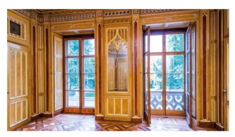
The front windows in the Château de l'Aile Vevey were reconstructed using thin SCHOTT RESTOVER® glass. The interior windows were also renovated using the original fittings.
