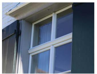
Dual-sash exterior windows installed with SCHOTT RESTOVER® insulating glass in the existing single-pane window casements.
