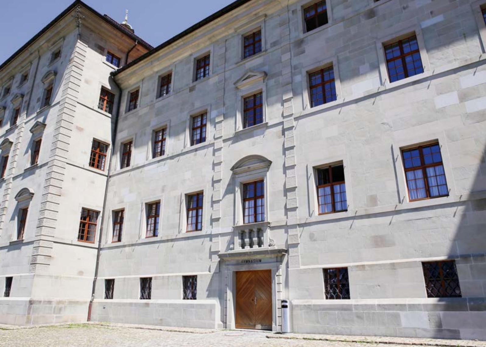
Full restoration is taking place from 2013 to 2022 and aims to recreate the original Baroque appearance which to some extent had been distorted by earlier renovations. The new renovation uses SCHOTT TIKANA® restoration glass in the main exterior of the Einsiedeln Abbey. The glass has a slightly irregular surface to blend harmoniously into the overall image, and combines a historical look with modern building properties.
