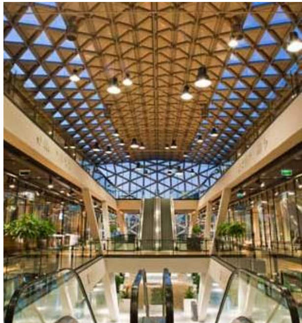
pic_10: The areas which cover escape routes, must meet fire protection requirements E (G) 30. This is where the specialty glass PYRAN® S from SCHOTT Technical Glass Solutions, Jena, was installed.
