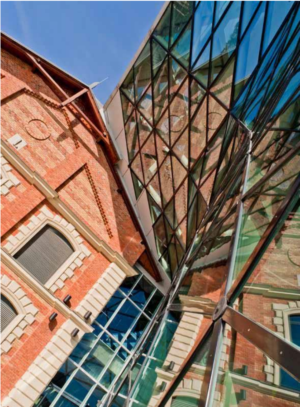
pic_01: Attractive mirroring effect at the connection between the landmarked warehouse and the new steel and glass structure.
