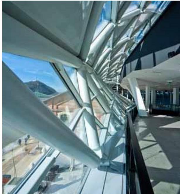
pic_08: The coated steel structure meets fire protection requirement E (G) 30.
