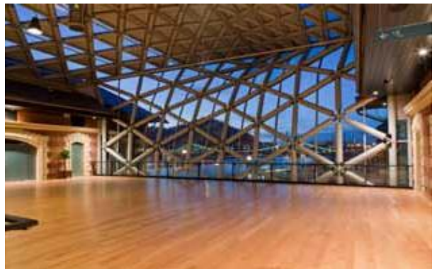
pic_06: A sophisticated design made of the specialty glass PYRAN® S from SCHOTT Technical Glass Solutions, Jena is part of the fire protection solution.
