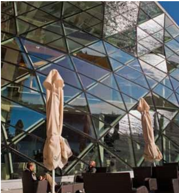
pic_09: The facade sections not located above escape routes are made of non-flammable materials. The Danube River is reflected in the large glass surfaces as it flows past.
