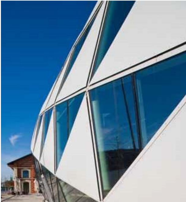
pic_07: The outside single walled covering was set directly onto the round steel pipes of the primary structure.
