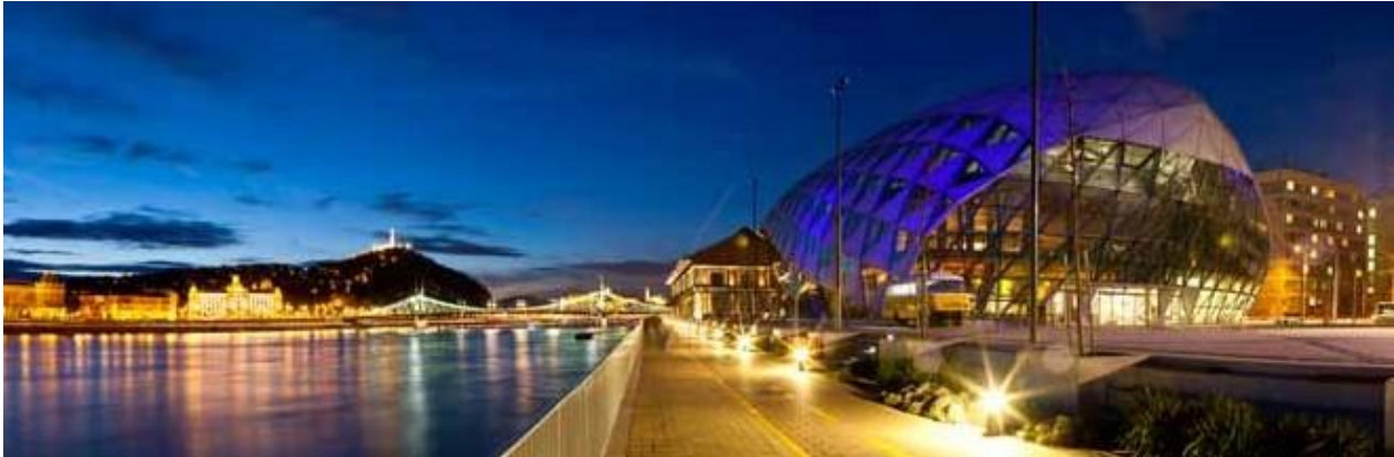
pic_02: In a prominent location in Budapest, the visionary structure enhances the skyline of this city on the Danube. The facade is constructed from a total of 405 large sized insulating glass elements made of the specialty glass PYRAN® S, alternating with triangular aluminium sandwich panels and glass elements with no fire resistant requirements.
