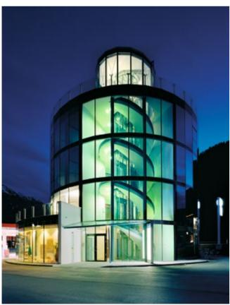
A frameless, point-supported glass facade was created for the Bluetower in St. Johann with SCHOTT fire resistant glazing. The connection of the double-glazed elements with PYRAN® S was achieved using purpose-built steel sections, which were attached with stainless steel point fittings at each intermediate floor.
