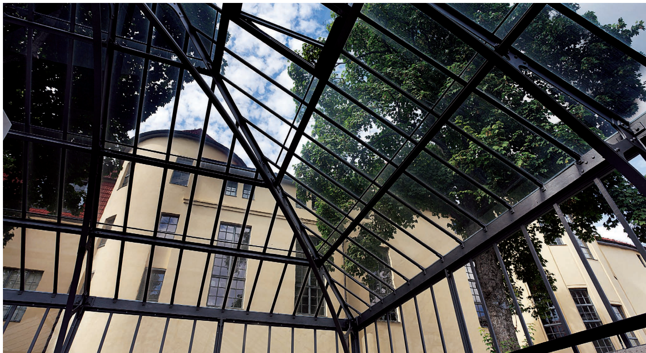
Bauhaus-University Weimar – The Brendel Studio using SCHOTT RESTOVER® laminated glass
