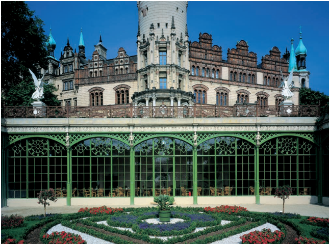
Orangery Schwerin Castle, Schwerin, Germany
