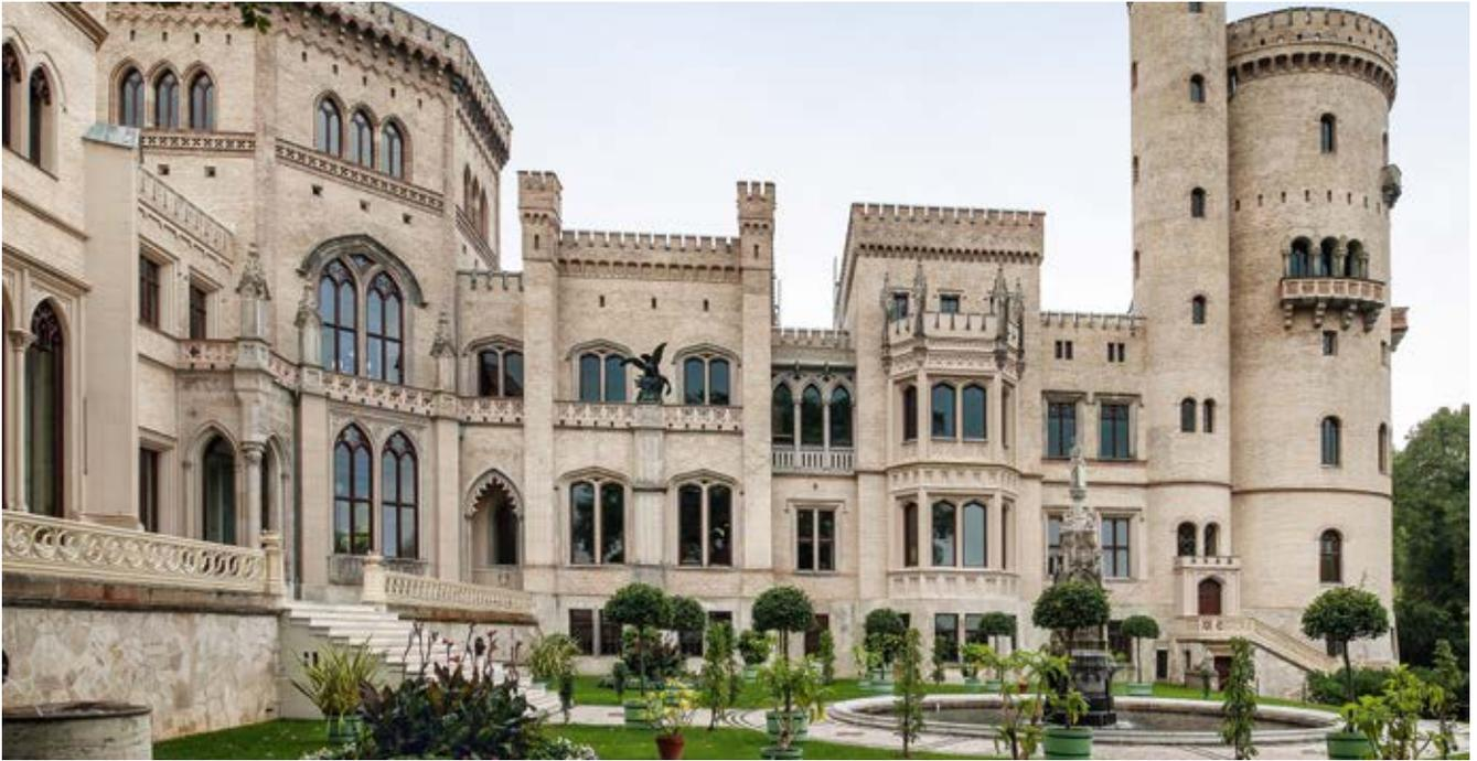
This allowed for a large share of the all glass windows to be installed. The 4.5 meter high special formats on the main floor of the palace were designed as laminated glass with butt joints. In addition, insulating glass with an outer pane made of GOETHEGLAS and an inner pane made of float glass was produced to address specific climatic concerns.
