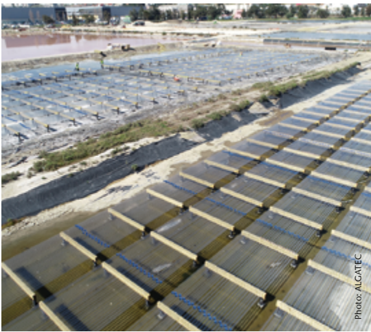
In the microalgae production systems at the ALGATEC Eco Business Park, A4F also uses tubular glass photobioreactors.
